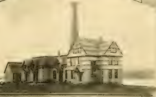
Water Works Pump House.
